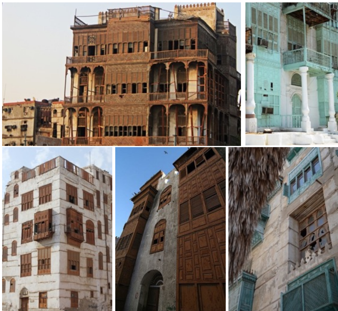
Figure 13 The "Musharabiyat" of old Jeddah, wooden elements covering windows and decorating the buildings in the Hijaz region. The green and turquoise colored "Roshan" are found on special buildings in Medina and Mecca
