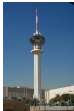
Figure 35 Saudi Television Tower
