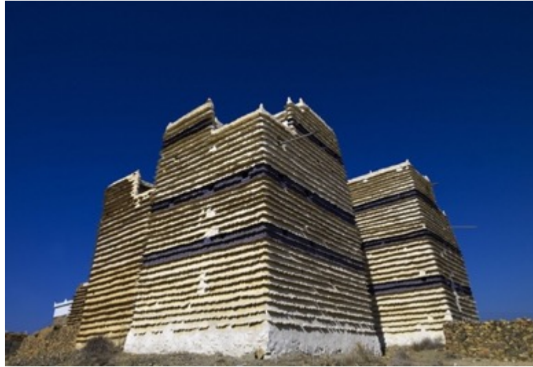
Figure 10 Houses in Khamis Mushayt with terraces. Asir Region south-west Saudi Arabia. Made of mud and stone to protect from the rain, the thick walls a keep the cool temperature during summer.
