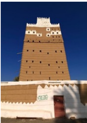
Figure 12 Traditional multi-storey adobe and brick house in Najran called a Midmakh building, it reflects the Yemeni influence in the province. Windows are smaller on lower floors for heat prevention and privacy, while on higher floors they are larger for air circulation and sunlight.
