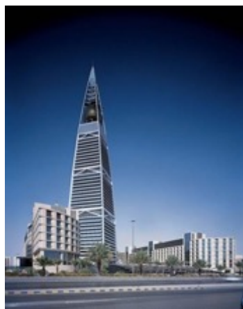
Figure 36 AlFaisaliah Tower and Commercial Centre
