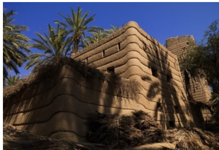
Figure 12 Traditional multi-storey adobe and brick house in Najran called a Midmakh building, it reflects the Yemeni influence in the province. Windows are smaller on lower floors for heat prevention and privacy, while on higher floors they are larger for air circulation and sunlight.
