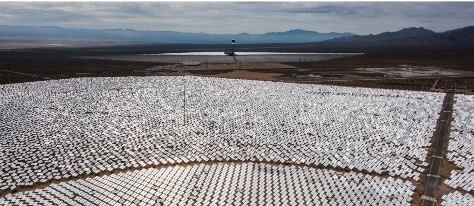
At the Ivanpah Solar Electric Generating System in California, 300,000 mirrors track the sun in two dimensions and reflect the sunlight to boilers atop three tall power towers. Photo by National Renewable Energy Lab (CC BY-NC-ND 2.0)
