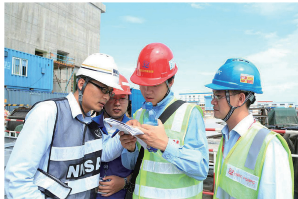
Fuqing NPP On-site Oversight by Inspectors from East China Regional Office of NNSA
