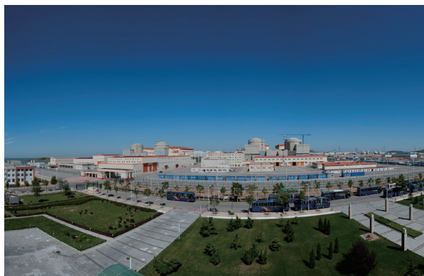
An Overall View of Hongyanhe NPP Phase I Unit 1 to Unit 4
