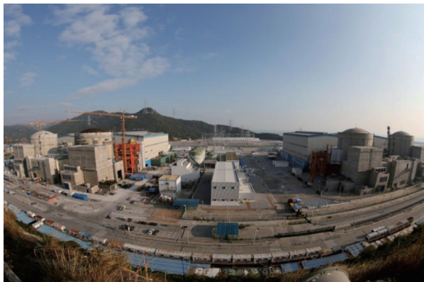
An Overall View of Yangjiang NPP Unit 1 to Unit 6
