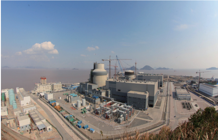
An Overall View of the Sanmen NPP Site
