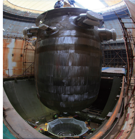
RPV Installation of Sanmen NPP Unit 2
