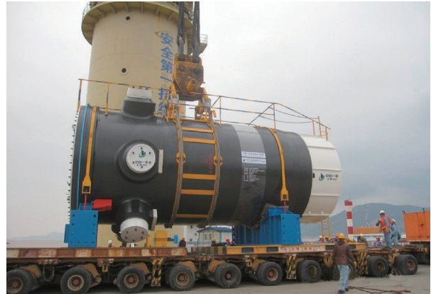
RPV of Ningde NPP Unit 4 Nuclear Island Arrived at the Site
