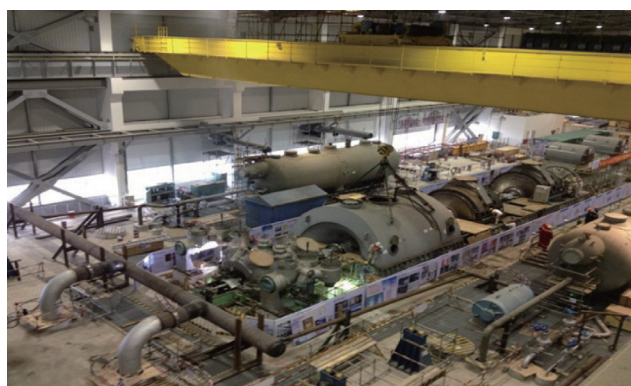
Installation of Hainan Changjiang NPP Unit 1 Steam Turbine
