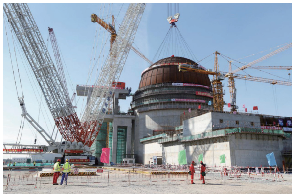
Hoisting of the Nuclear Island Containment Dome of Tianwan NPP unit 3
