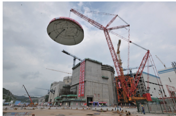
Dome Hoisting of Yangjiang Unit 4
