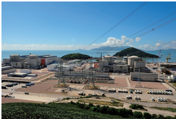
An Overall View of Ningde NPP Unit 1 to Unit 4
