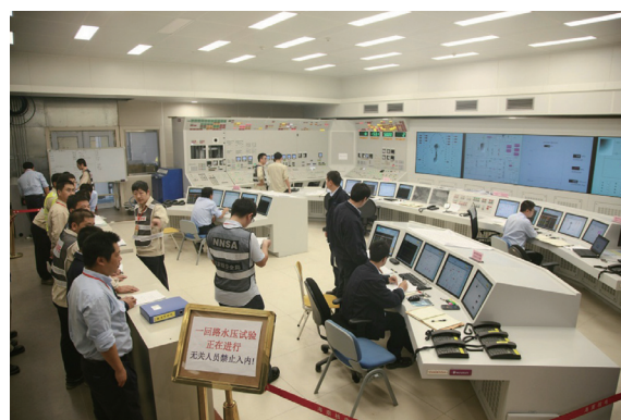
Oversight of Primary Loop Hydro Test on Hainan Changjiang NPP Unit 1
