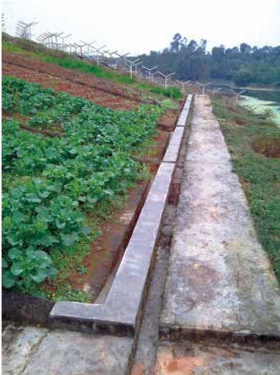
Rainwater harvesting ditch
