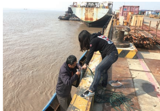
Maintenance of water monitoring devices of the Yangtze River
