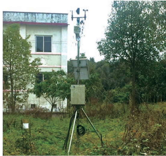
Automatic meteorological observation station
