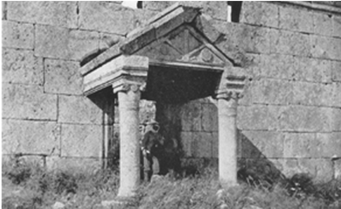
Fig. 2: Bātūta (5 th century A.D.), pediment of porch with a bas-relief representing a king post truss where the post is mortised into the tie-beam (Butler 1929, p. 201).
