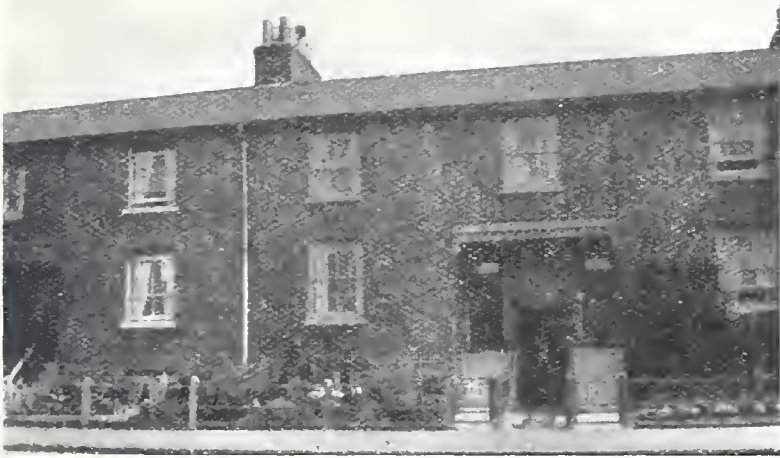
Steps. Tunnel through house.
