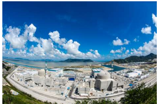
Figure 15. Complete view of Taishan NPP
