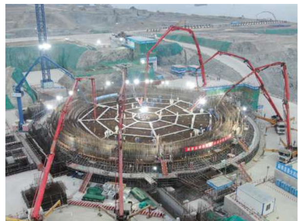
Figure 20. Concrete casting site of Taipingling NPP Unit 1
