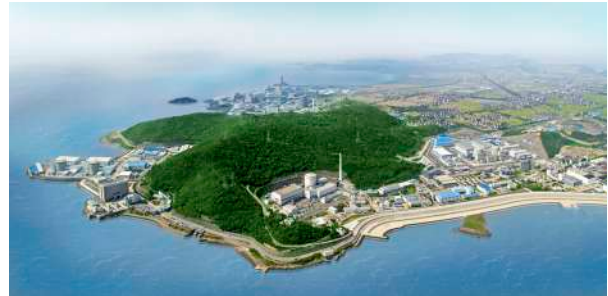
Figure 1. Complete view of the Qinshan Nuclear Power Base
