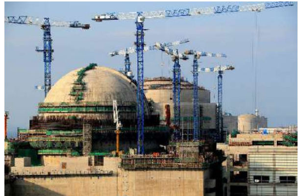
Figure 9. Construction site of Fuqing NPP Units 5 and 6
