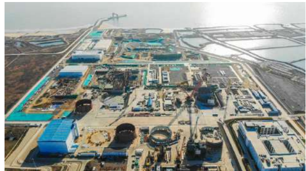
Figure 17. Construction site of National Nuclear Demonstration Project
