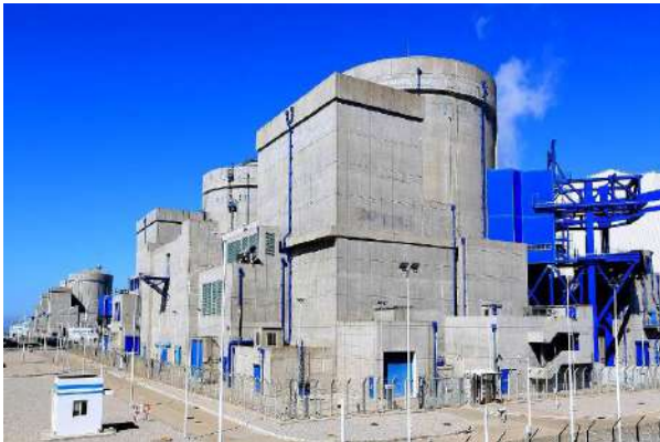
Figure 8. Fuqing NPP Units 1-4
