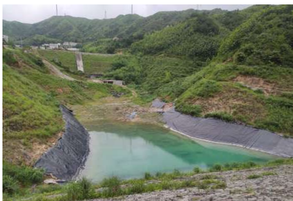
Figure 23. Anti-seepage facilities of the mill tailing repository
