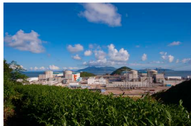
Figure 7. Ningde NPP Units 1-4
