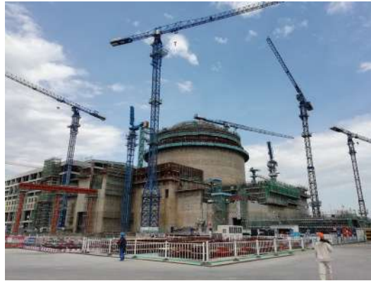
Figure 12. Construction site of Fangchenggang NPP Unit 3 Project
