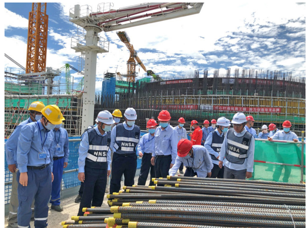
Figure 9. Inspectors Inspecting at the Site of Changjiang NPP
