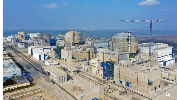
Figure 8. Units 1 to 6 of Fuqing NPP
