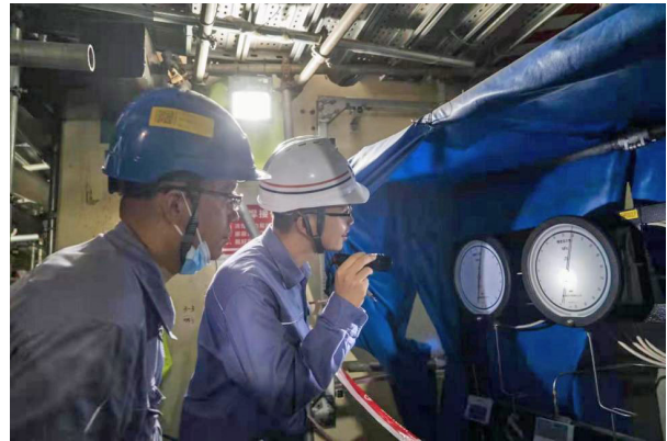
Figure 10. Cold Test Site of Unit 3 of Fangchenggang NPP
