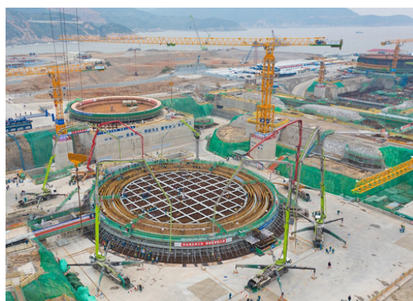
Figure 17. Concrete Pouring Site of San'ao NPP Unit 2
