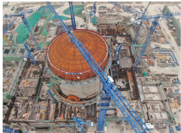
Figure 16. Construction Site of Taipingling NPP Unit 1
