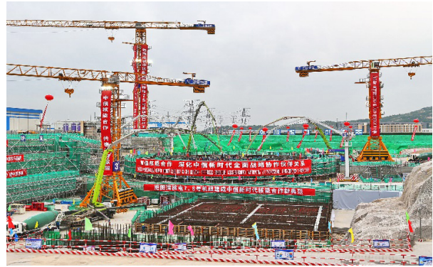
Figure 4. Construction Site of Tianwan NPP Unit 7
