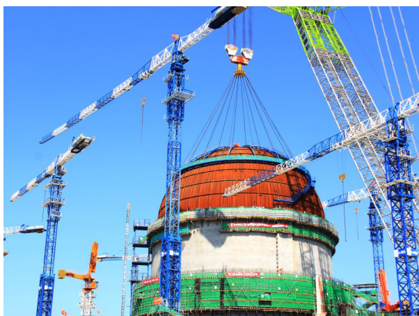
Figure 14. Dome Installation of Zhangzhou Unit 1
