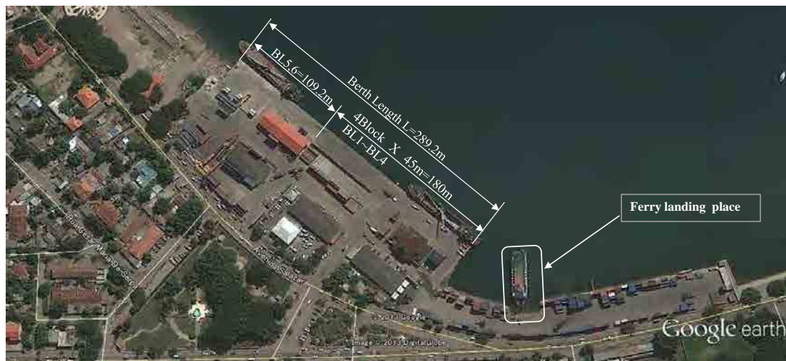
Figure 1.2-1 Mooring Facilities of Dili Port
