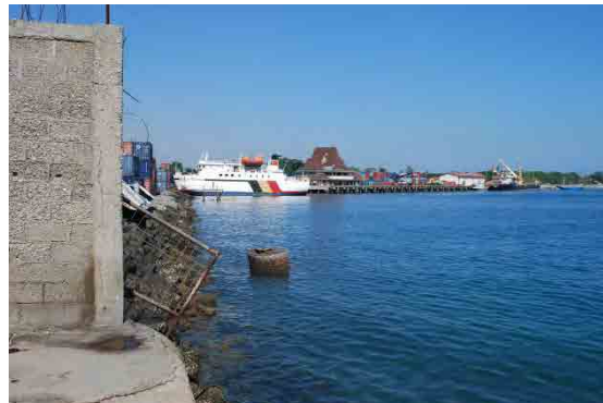
Figure 1.6-8 East Fence Seaside Edge
