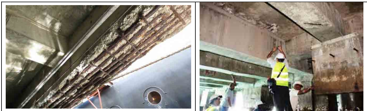
Figure 5.2-1 Inspection of Deterioration on BL5 and BL6
