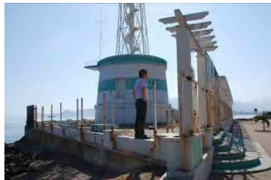
Figure 1.6-15 Fence of Lighthouse
