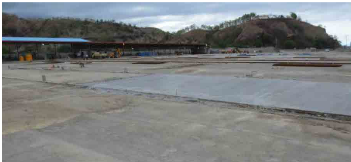
Figure 1.2-9 Dry Port under construction at Tasitolu (as of November 2013 )
