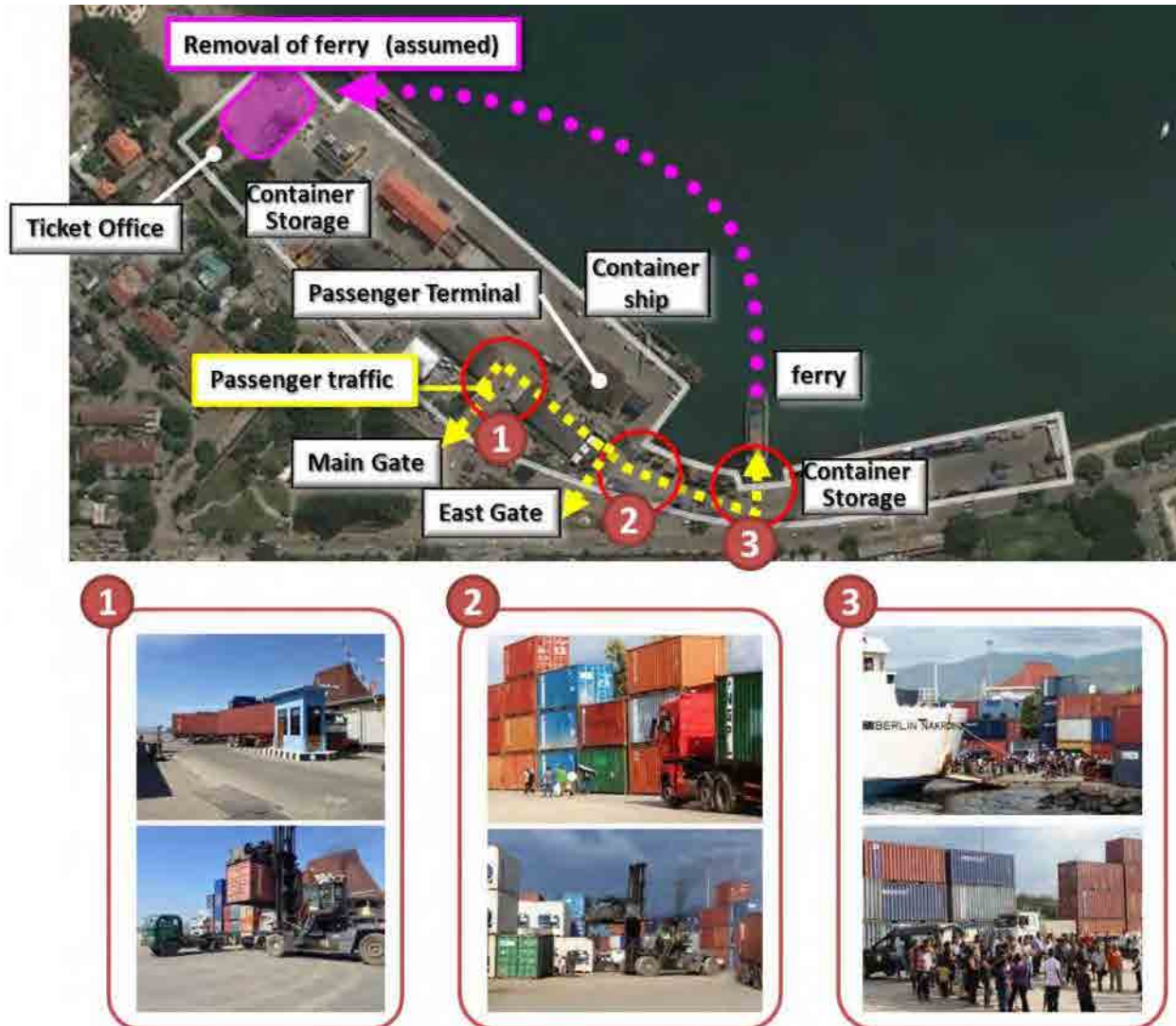
Figure 6.2-1 Problems on Passenger Handling and Relocation of the Ferry to West Side
