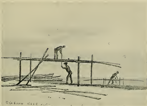
RIPPING TIMBERS FOR THE SCHOONER
