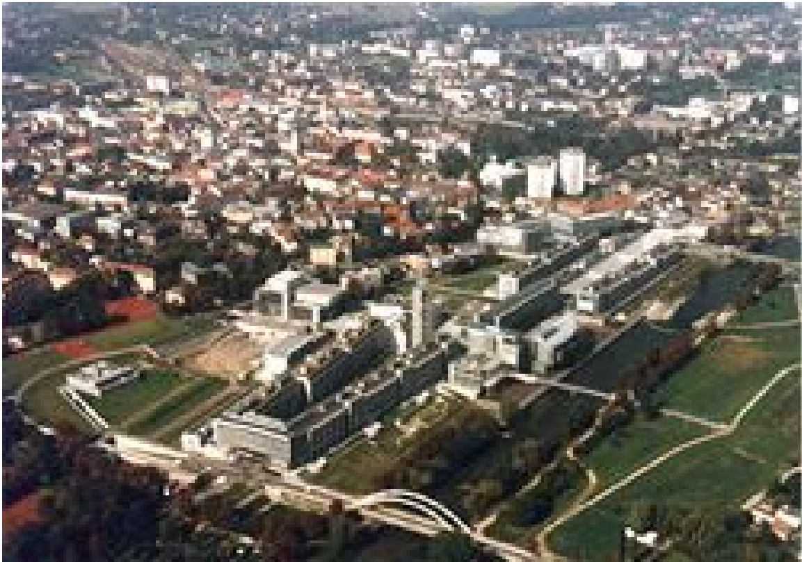
Figure 11 Aerial view of St. Pölten
