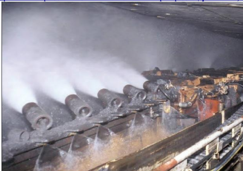
Figure 3-8.—Venturi sprays mounted on headgate splitter arm.
