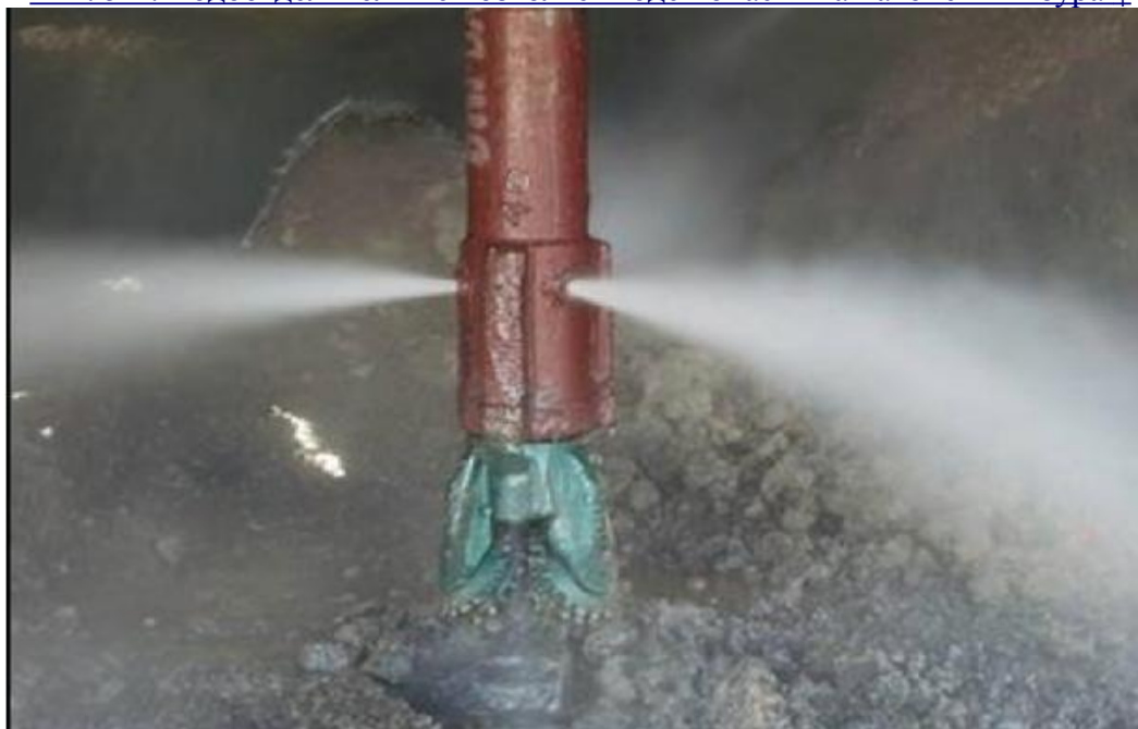
Figure 5-2.—Water separator discharging water before it reaches the drill bit.
