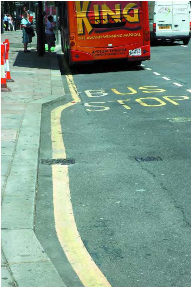
Partial build-out within bus bay
