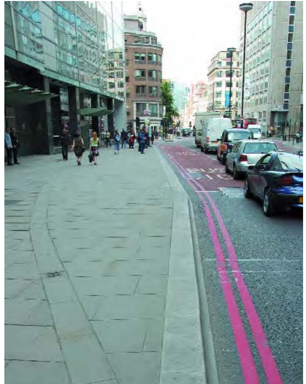
Fully filled bus bay
