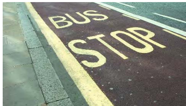
Clearway marking – Borough controlled road
