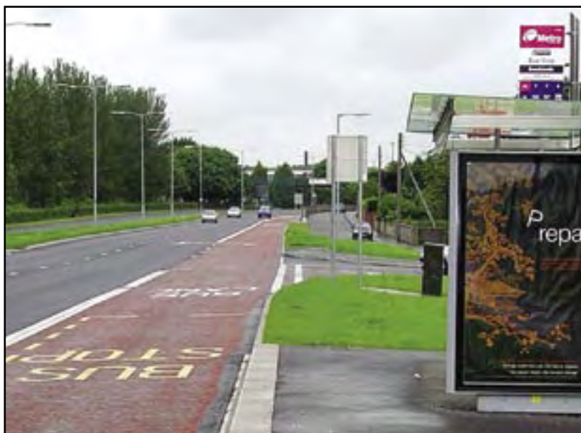
Photo 7c – Easy access kerbs used in bus boarder
