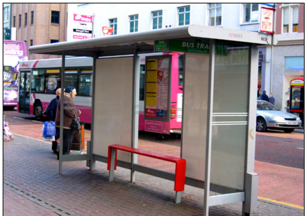
Photo 6h - Typical shelter with perch seat
