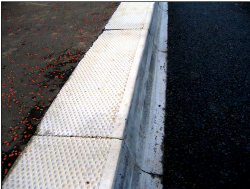
Photo 7g – Close-up of easy access kerbing
