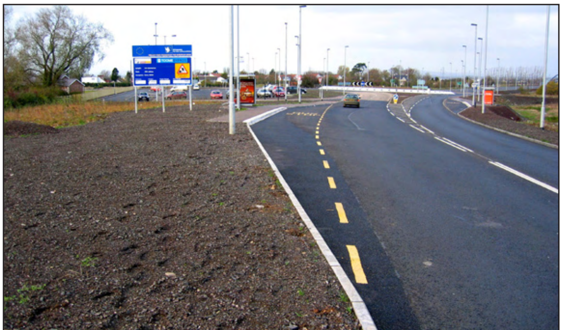
Photo 8k - Typical lay-by – Toome Bypass
