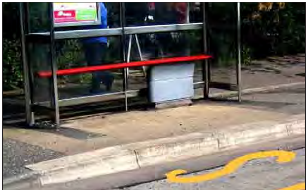
Photo 7c – Easy access kerbs used in bus boarder
