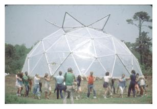
When the I pillows are inflated, the entire dome is put under compressive load that tends to oppose the considerable wind lift, This preloading, together with the anchoring provided by buried concrete blocks tied to the lowest hubs, has withstood 30 inches of snow load and winds well above 100 mph. This may be considered good performance from a structure that weighs but 1/2 lb/ft2 of floorspace (less than 500 lbs total). The light weight not only results in low shipping
