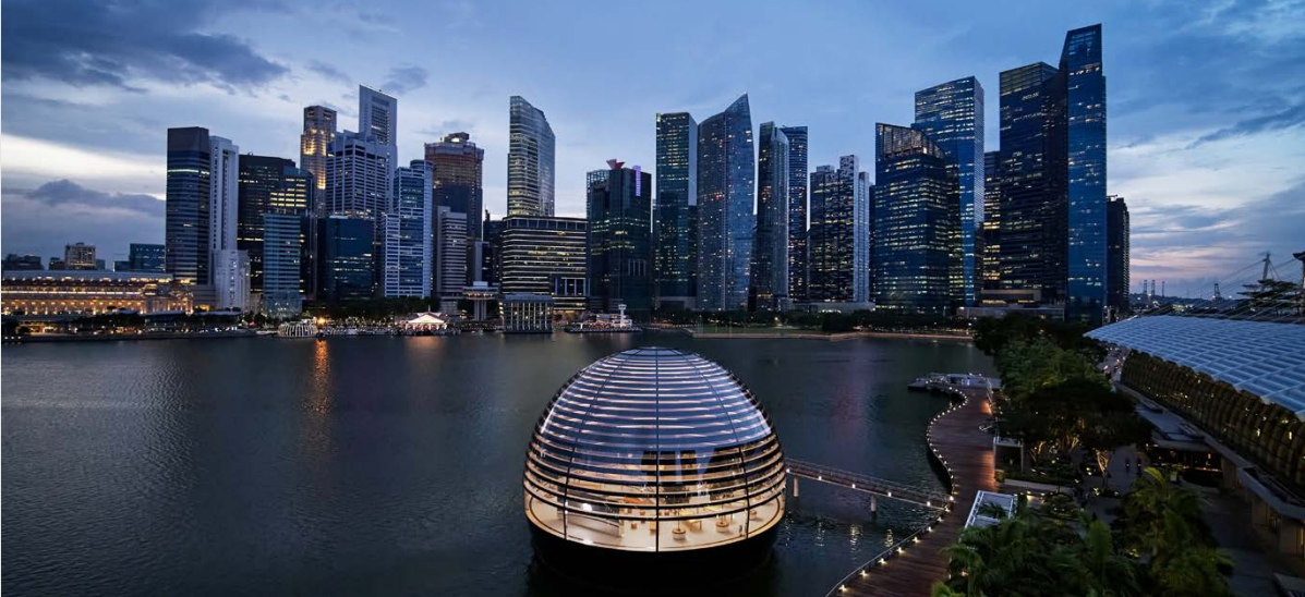
Left: Our Marina Bay Sands retail store in Singapore features energy-efficient design and FSC-certified wood.
