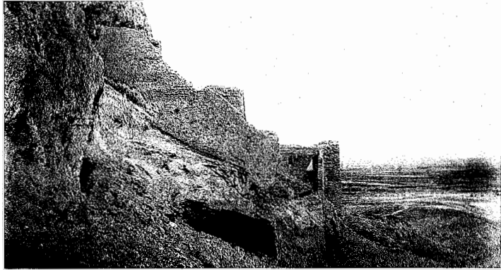
DEIR BALYZEH, SOUTH OUTER WALL.
