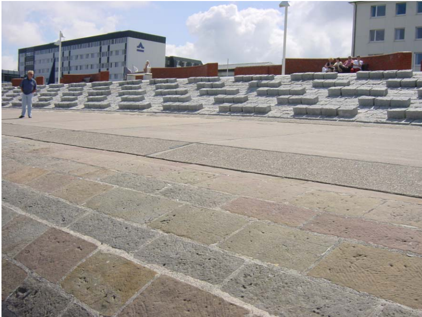
Figure 5.19: Example for roughness elements (photo: Schüttrumpf)
