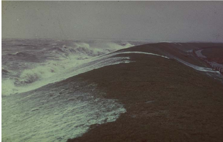
Figure 5.23: Short crested waves resulting in wave run-up and wave overtopping (photo: Zitscher)
