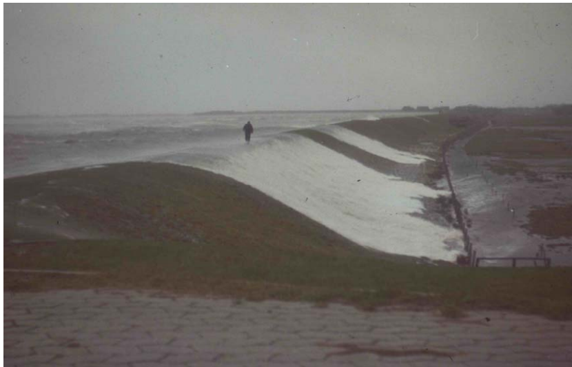
Figure 5.33: Wave overtopping on the landward side of a seadike (photo: Zitscher)
