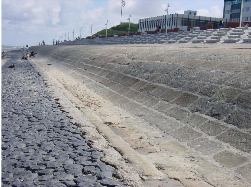
Figure 5.17: Dike covered by natural bloc revetment (photo: Schüttrumpf)
