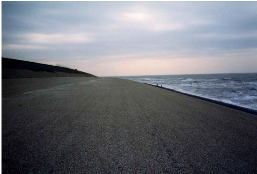
Figure 5.16: Dike covered by asphalt (photo: Schüttrumpf)
