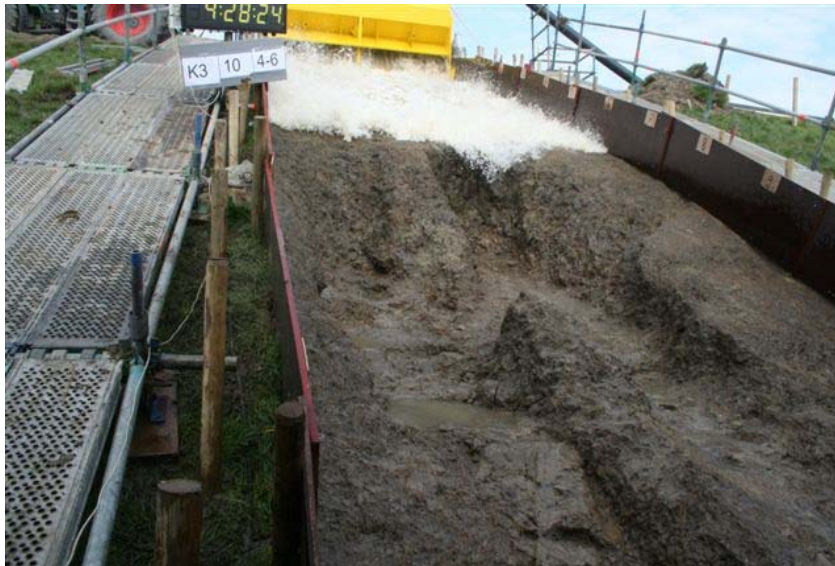
Figure 3.2: Wave overtopping test on bare clay; result after 6 hours with 10 l/s per m width
