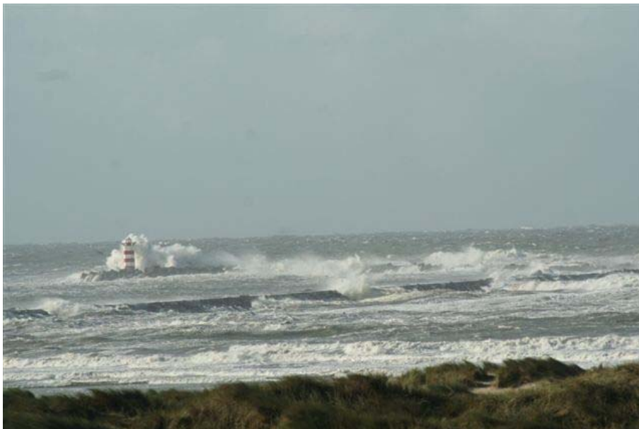
Figure 4.10: Wave overtopping and transmission at breakwater IJmuiden, the Netherlands
