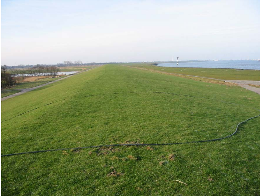
Figure 5.15: Dike covered by grass (photo: Schüttrumpf)
