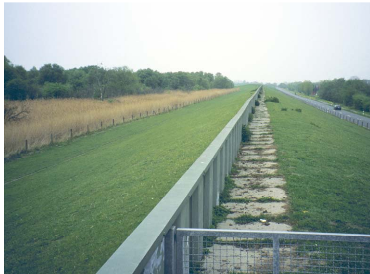
Figure 5.30: Sea dike with vertical crest wall (photo: Hofstede)
