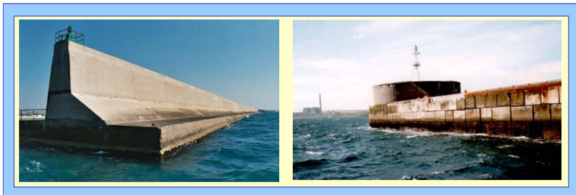
Figure 7.1: Examples of vertical breakwaters: (left) modern concrete caisson and (right) older structure constructed from concrete blocks
