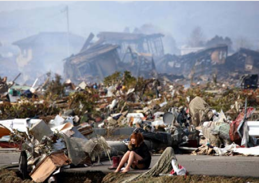
The toll of the 2011 great Tohoku earthquake and tsunami in Natori city, Japan, where more than 900 people were reported dead.
