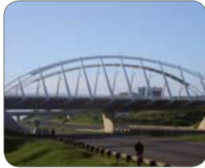
Grade 1.4003/410 painted, SASSDA, South Africa (bridge in service for over 8 years).
