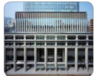
Outer parts SUS445J1, inner SUS304, Nihonbashi Mitsui Bldg., 2005, Japan
