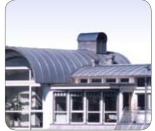
Grade 430Ti (standing seam technique), Ugine & Alz, Austria
