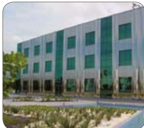
Grade 1.4521/444 brushed no. 4 (horizontal panels), Vivo Building, Rio de Janeiro, Nucleo Inox, Brazil (coastal environment)
