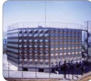
Partially in grade SUS444, finish no. 4, JSSA, Japan
