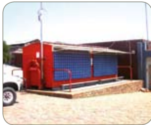
Grade 1.4003/410, painted, SASSDA, South Africa. "Utility" ferritics are often painted, when aesthetic considerations are important.
