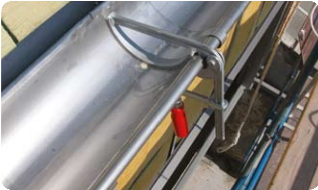
Bonding of guttering, tin-coated 430Ti.
