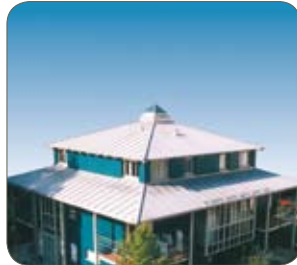
Grade 1.4510/430Ti (standing-seam technique), Ugine & Alz, Germany.
