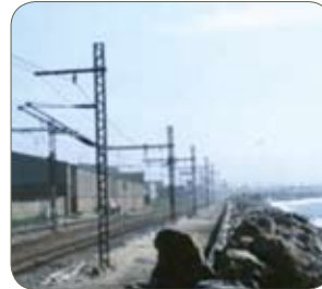
Grade 1.4003 (first major application in 1982, along seashore – 10m from surf, no corrosion), S. Africa
