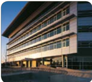
Grade SUS445M2, low-reflectivity matt finish, ASSDA, Australia
