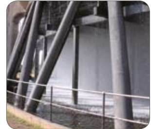
Grade 1.4003/ 410, X-grid cooling tower packing, S. Africa
