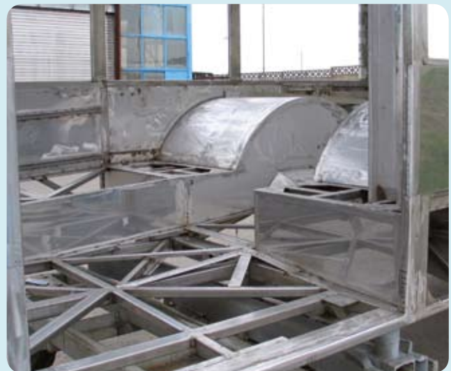
Welded structural frame in grade 1.4003.
