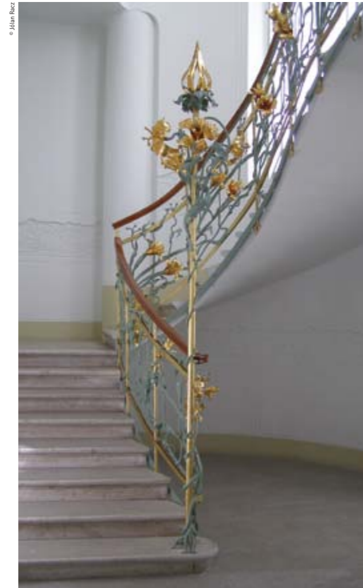
Wrought iron balustrade by Pl Fekete, after drawings by architect Ede Magyar
