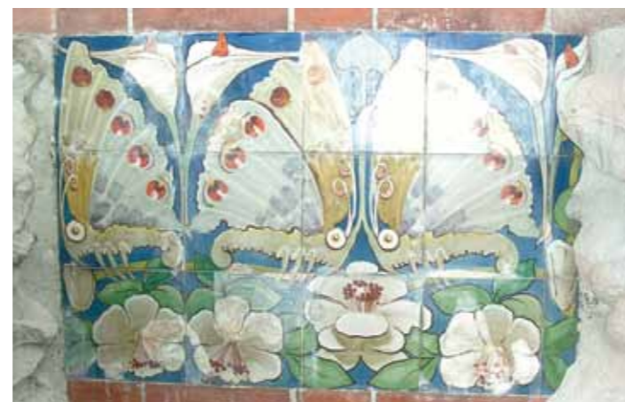
Detail of façade frieze at the height of the first floor, made with ceramic tiles representing a series of silkmoths
