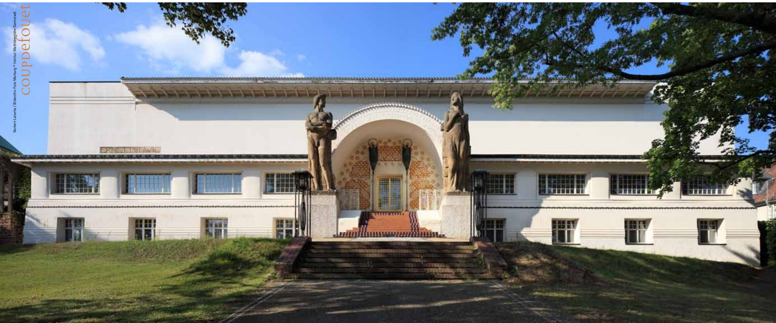
Main façade of the Ernst Ludwig House. Built in 1901 by Joseph Maria Olbrich, it was restored in the 1980s and has housed the Artists' Colony Museum since 1990
