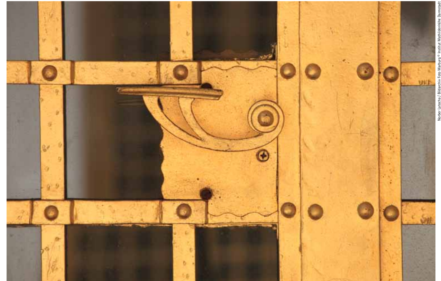
Detail of the original south entrance door of the Ernst Ludwig House, designed by Joseph Maria Olbrich, 1901 Detall de la porta de l'entrada sud original de la Casa Ernst Ludwig, dissenyada per Joseph Maria Olbrich, 1901
