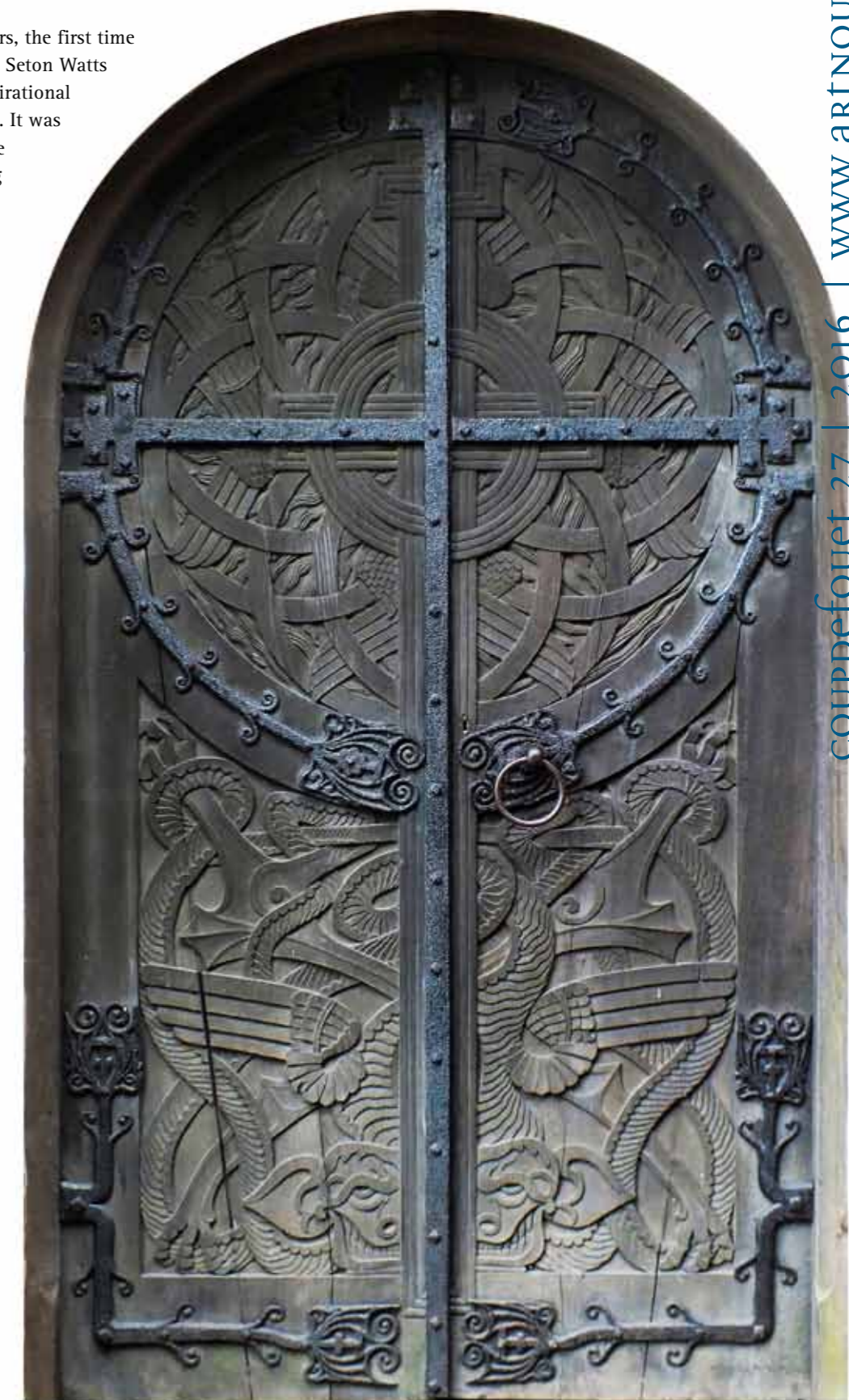
Entrance door, with symbols of light in the top circle and of the defeated dragon below. Ironwork designed by George Redmayne
