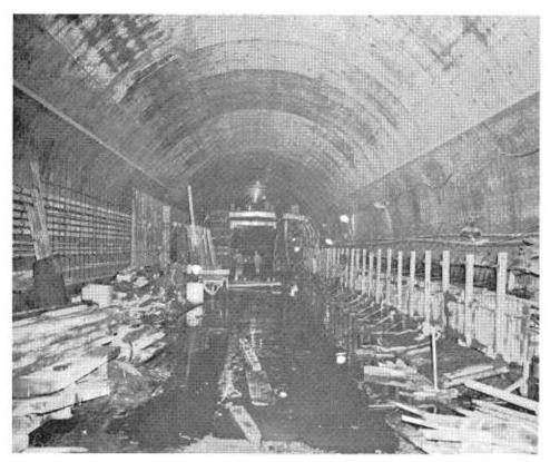
The subway interior work in progress with the wall, walk and ceiling forms in place. The 10 ducts inside the wall form are for telephone cables. Note the limited working space and the difficult access conditions.
