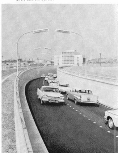
Other "vital statistics" include: tube segments, total of 12, each weighing 11,000,000 pounds; 67,000 cubic yards of concrete; maximum roadway depth, 72 feet below mean sea level; length, including approaches, 5,923 feet; roadway width, 24 feet; vertical clearance, 15 feet.
