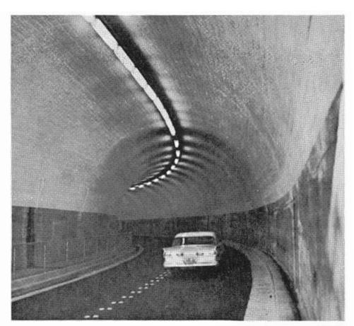
NOW. Interior view of tunnel, December 1962. Note the use of reflectorized buttons, fluorescent lighting fixtures and pedestrian protection fence.
