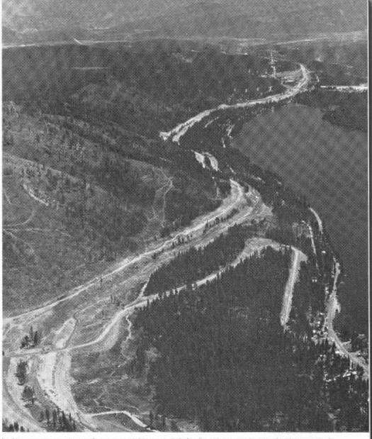
Looking east in reverse to photo on opposite page. Split-level roadways climb side of ridge on steady, easy grade, eliminating steep, tortuous climb up east face of Donner. Additional lane will be provided on upgrade roadways for slow-moving vehicles.
