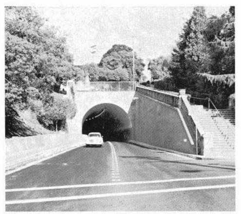
NOW. Southerly end of Solano Avenue project at Sutter Street. The raised reflectorized buttons have proved effective in channeling traffic into the proper lane. Note extensive landscaping.
