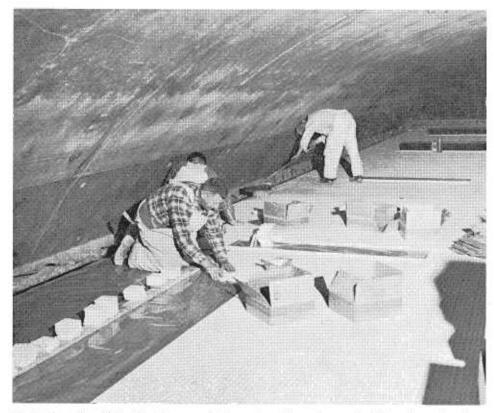
Placing the ceiling tile in the tube segments from above. Gummed paper is laid on the ceiling form, the paper moistened, and the tile placed face down on the paper. Next, the slab reinforcing steel is placed and then the concrete, including an inch of grout cover over the tile. The paper is then removed, exposing the tile.
