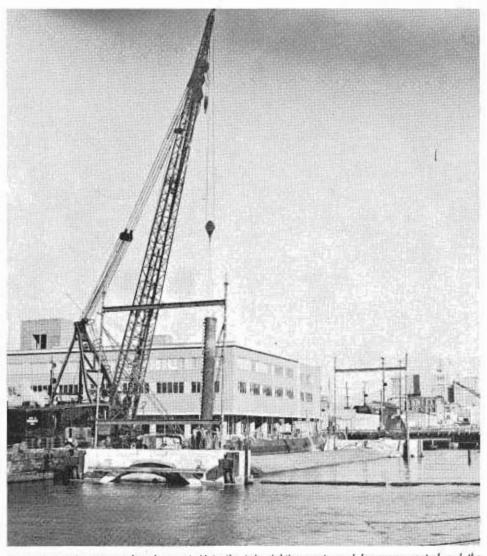
Preparing a tube segment for placement. Note the twin sighting masts used for survey control and the manhole used for access and ventilation being lowered into position by the crane.
