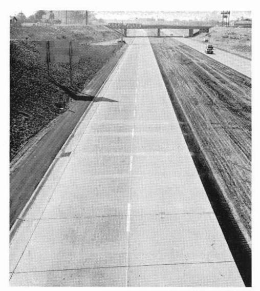
Newport Freeway in Orange County, shown above from an overcrossing and below from the air, was chosen for tests because it was new, and also had very good profile index. Joints show clearly in above photo; scene is close to junction with Santa Ana Freeway, intersection with which shows in aerial.
