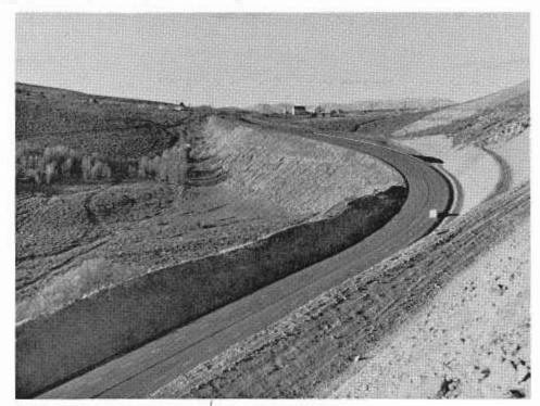
A section of the new highway over the 8,136-foot-high Conway Summit. Note the southwest cuts on the left laid back for maximum exposure to the sun.
