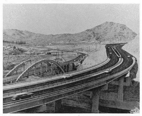
The Mojave River Bridge and Overhead at Victorville Narrows, looking eastward. The recently completed bridge carrying Sign Route 18 traffic is on the right. The old arch bridge on the left now serves as a haul road for ore trucks to a lime rock products plant.
