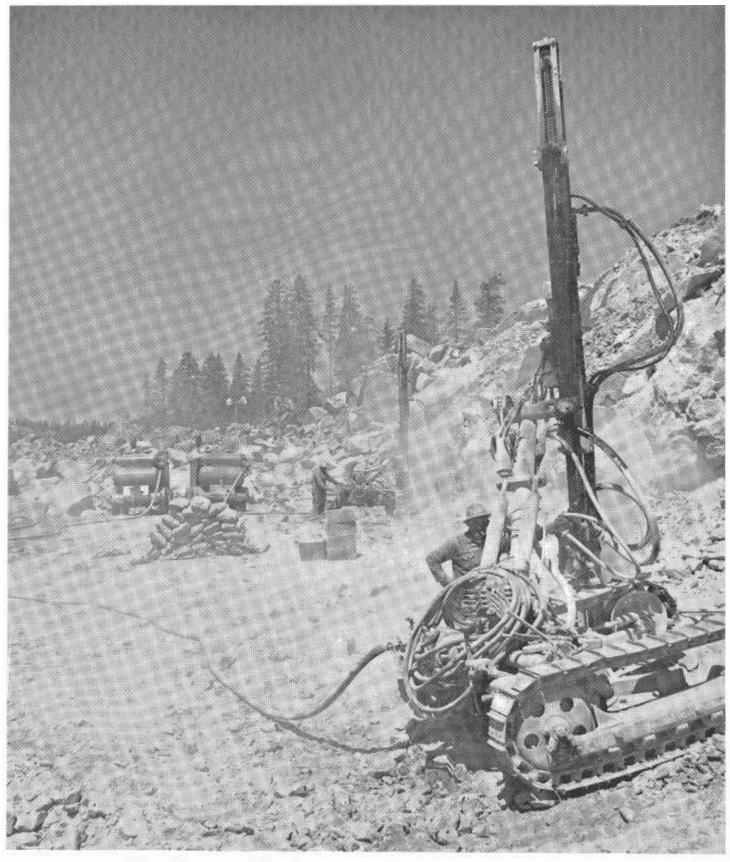
Self-propelled pneumatic drills here shown in operation have been used in dozens of places on summit jobs to build road through sheer granite.
