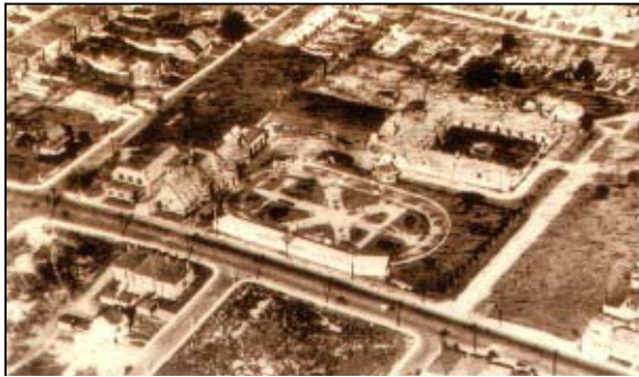
Aerial view of the RCAF Institute of Aviation Medicine site.
