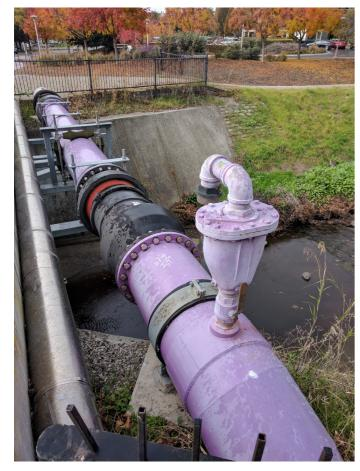
A lavender-colored pipeline carrying nonpotable water in a dual piping system in Mountain View, California. *Photo: Grendelkhan, CC BY-SA 3.0*
