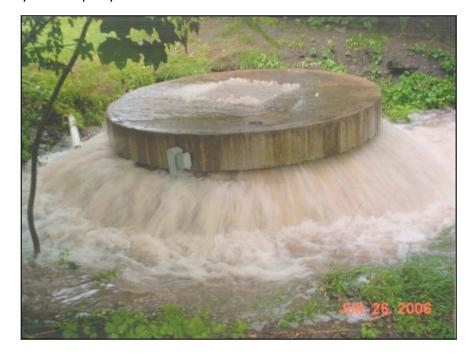
Figure. A combined sewer overflow event discharging excess sanitary and storm water. For scale, the circular vault cap is approximately 6-feet in diameter.
