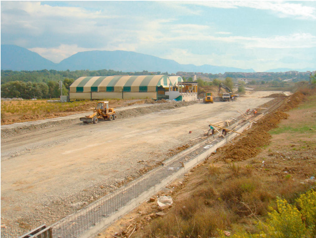
Photo 2.1: Highway construction in Tirana
