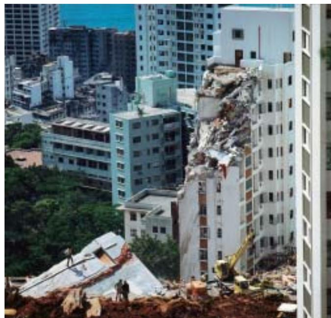
Fig. 2.52 Only half of another building on Kotewall Road remained intact after being struck by the toppled building higher up the slope (18 June 1972). Courtesy Hong Kong SAR Information Services Department
