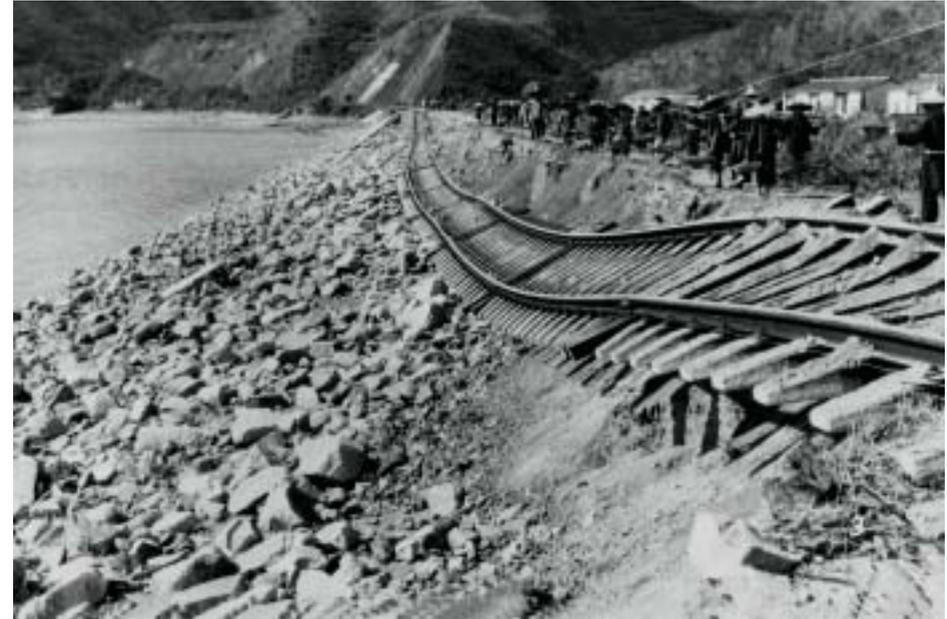
Fig. 2.5 A typhoon struck in September 1937, causing the loss of more than 11,000 lives. The Kowloon – Canton Railway track at Sha Tin was damaged during the typhoon. Courtesy Hong Kong SAR Public Records Office
