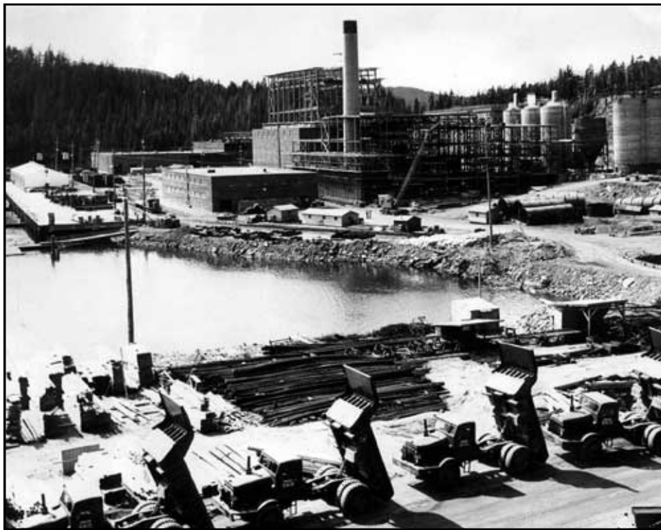
Ketchikan Pulp Mill construction, 1953
