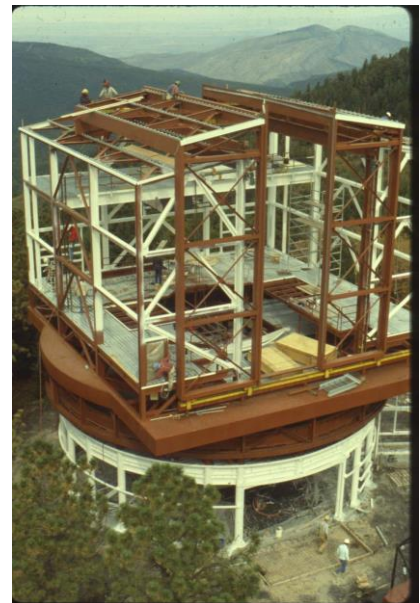
Figure 7 - 3.5 m telescope enclosure under construction. Courtesy of ARC.
