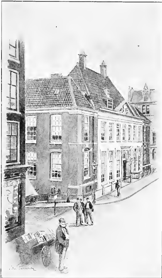
DUTCH WEST INDIA COMPANY'S HOUSE, HAARLEM STREET, AMSTERDAM
