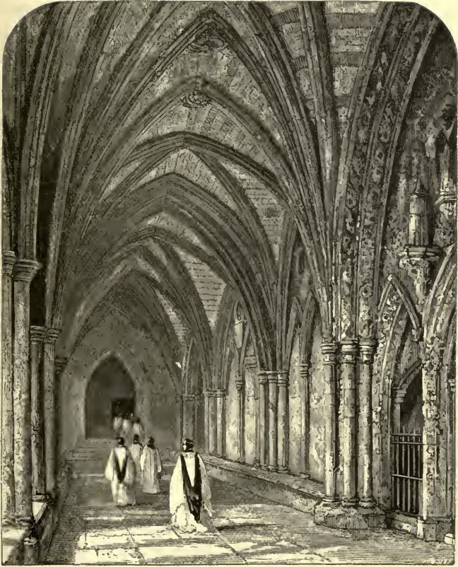
THE CLOISTERS, WITH ENTRANCE TO THE CHAPTER HOUSE.
