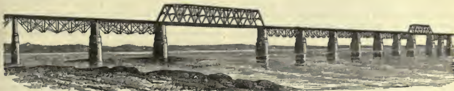
VIADUCT BRIDGE AT LOUISVILLE.
