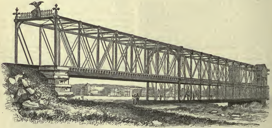
TRUSS BRIDGE OVER THE MISSISSIPPI BETWEEN DAVENPORT (IOWA) AND ROCK ISLAND (ILLINOIS).
