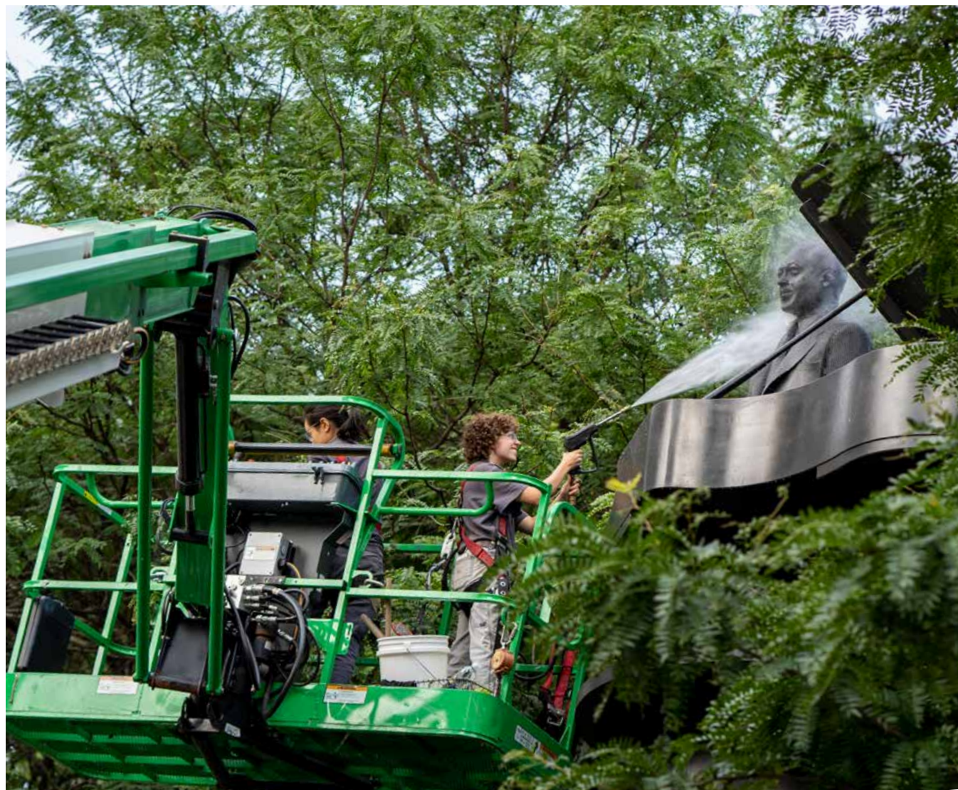
Monuments Conservation Technician Interns Hillary Gao and Isabelle Lobley use a power washer to clean the Duke Ellington statue.
