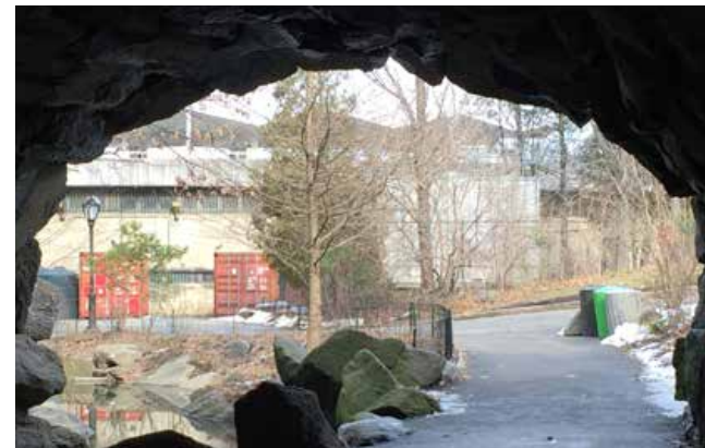
Existing view through Huddleston Arch
