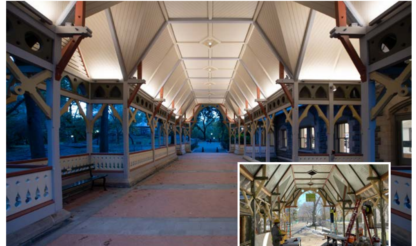
The historic loggia, pictured here post-restoration, was repaired as part of the comprehensive renovation; inset: construction underway.
