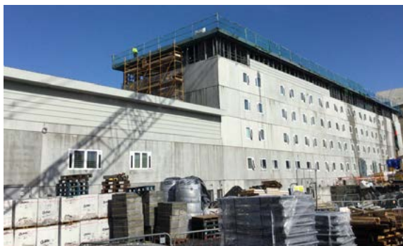
New FSI Laboratory under construction, Backweston, Co-Kildare
