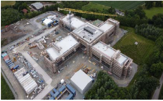
New FSI Laboratory under construction at Backweston, Co. Kildare
