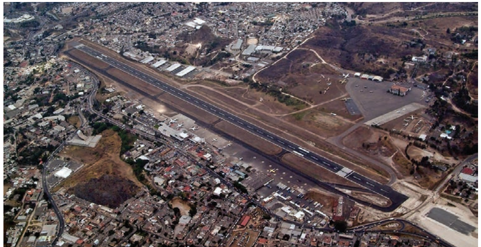
Tegucigalpa's runway has been lengthened to a safer 6,631 feet.
