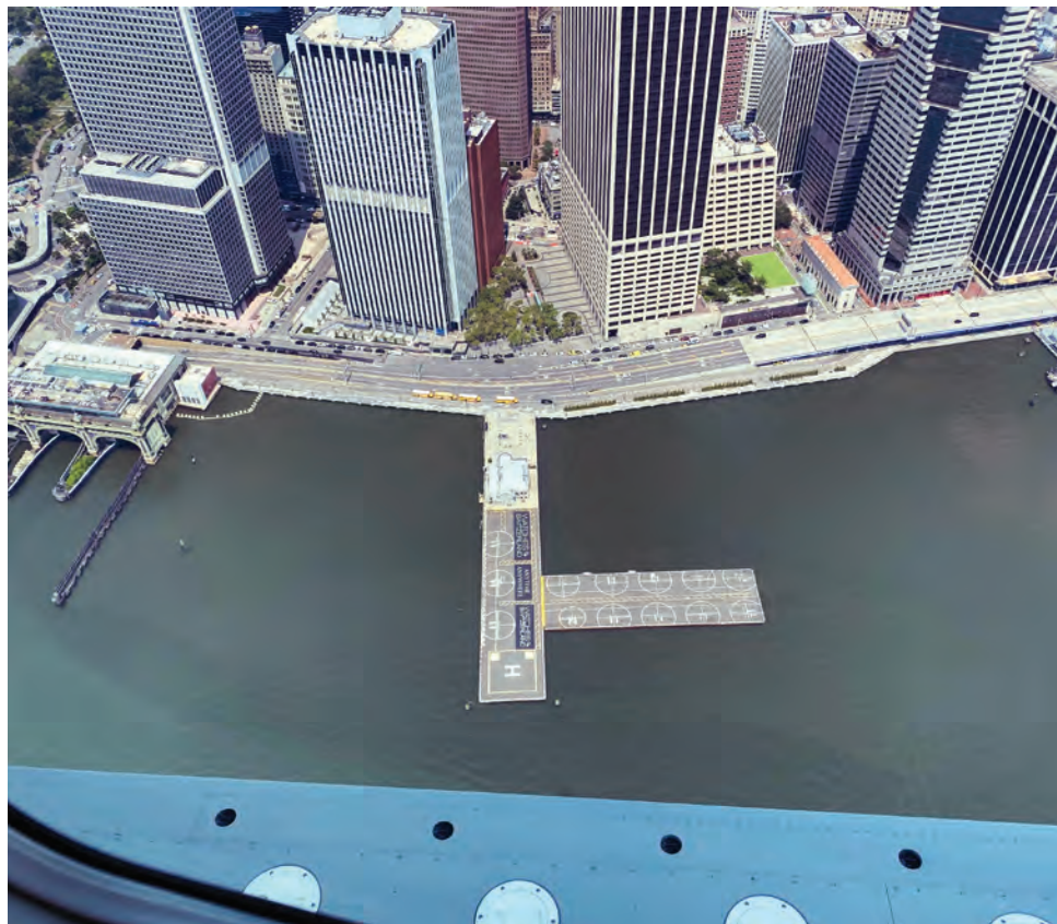
Well-designed heliports like New York City's Wall Street facility, are the exception, not the rule.
