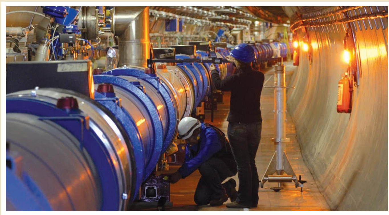
March: Precision is the name of the game as, once in position in the tunnel, the LHC's magnets are carefully aligned.
