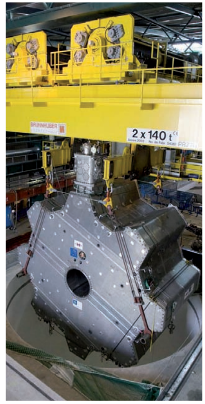
Lowering the second ATLAS endcap toroid magnet into the cavern in July.
