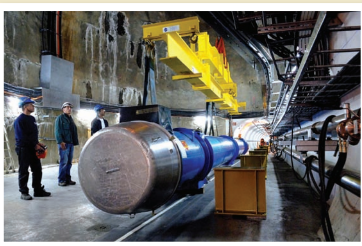
The last of 1746 superconducting magnets is lowered into the LHC tunnel via a specially constructed pit at 12.00 on 26 April. This 15 m long dipole magnet is one of 1232 dipoles that will guide the two proton beams in opposite directions around the 27 km circumference.
