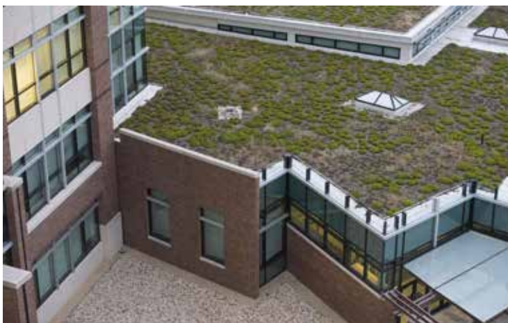
Figure 9.4: Living roof on a building at the US Air Force Joint Base Andrews, MD.
