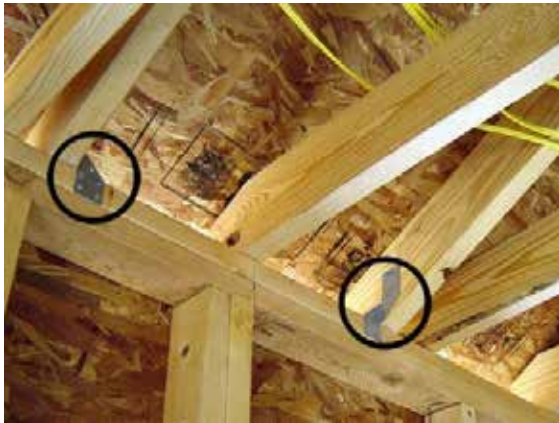
Figure 9.8: Hurricane clips, shown circled above, help anchor roofs to the main structure to prevent detachment due to severe wind. These clips can be found at many hardware stores, and are an inexpensive way to mitigate home damage from hurricanes. The home above kept its lid on during the severe winds brought by Hurricane Katrina, even though construction of the house had not been completed.
