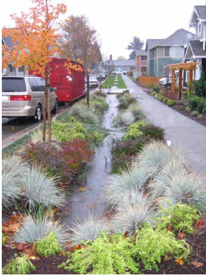
Figure 9.6: Rain garden in the High Point neighborhood in Seattle, WA.
