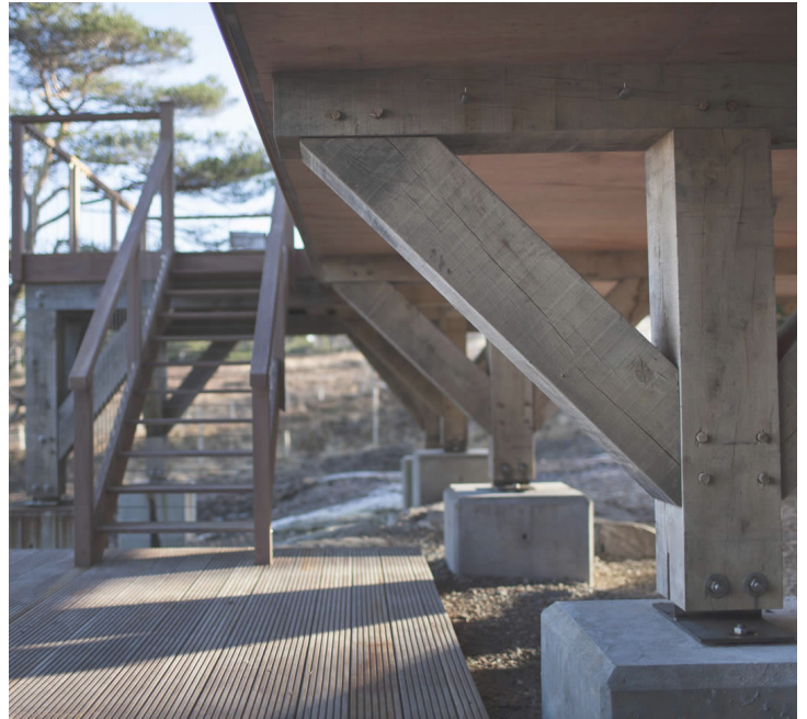
figure 16: external timber deck
