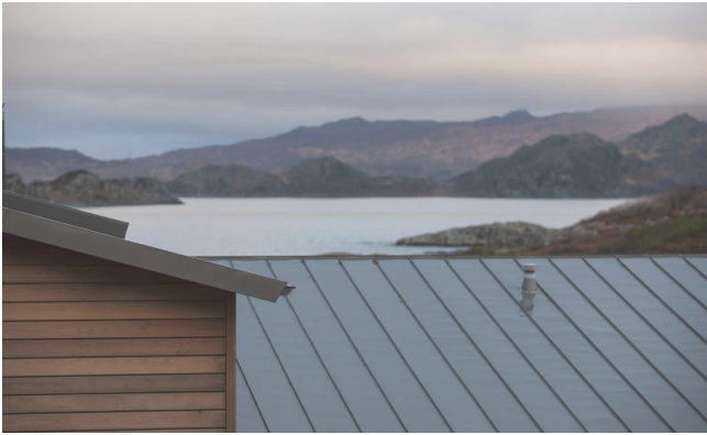
figure 13: standing seam zinc (cladding and roofing)
