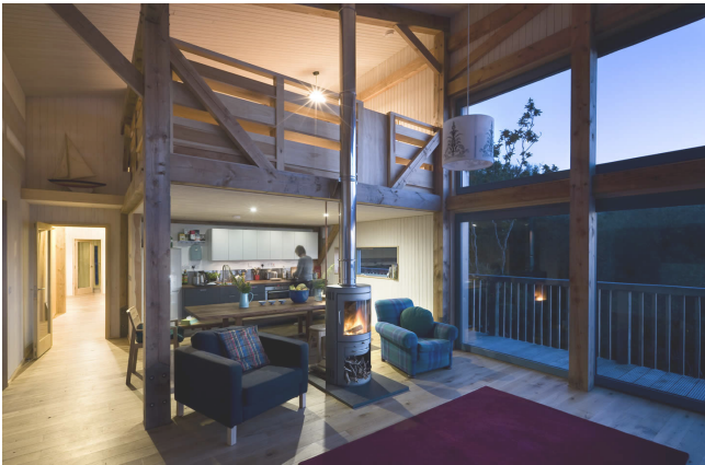
figure 15: expressed timber internal structure
