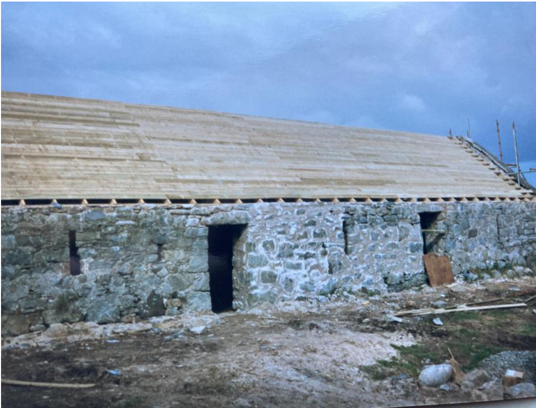
Image 11b – Example of rebuilt and repointed walls (1999 Works)
