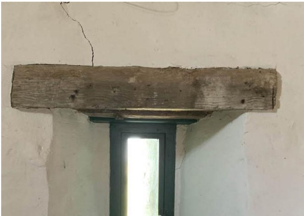
Image 18 – Example of timber lintel
