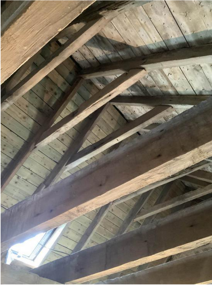
Image 12 – Example of roof timbers
