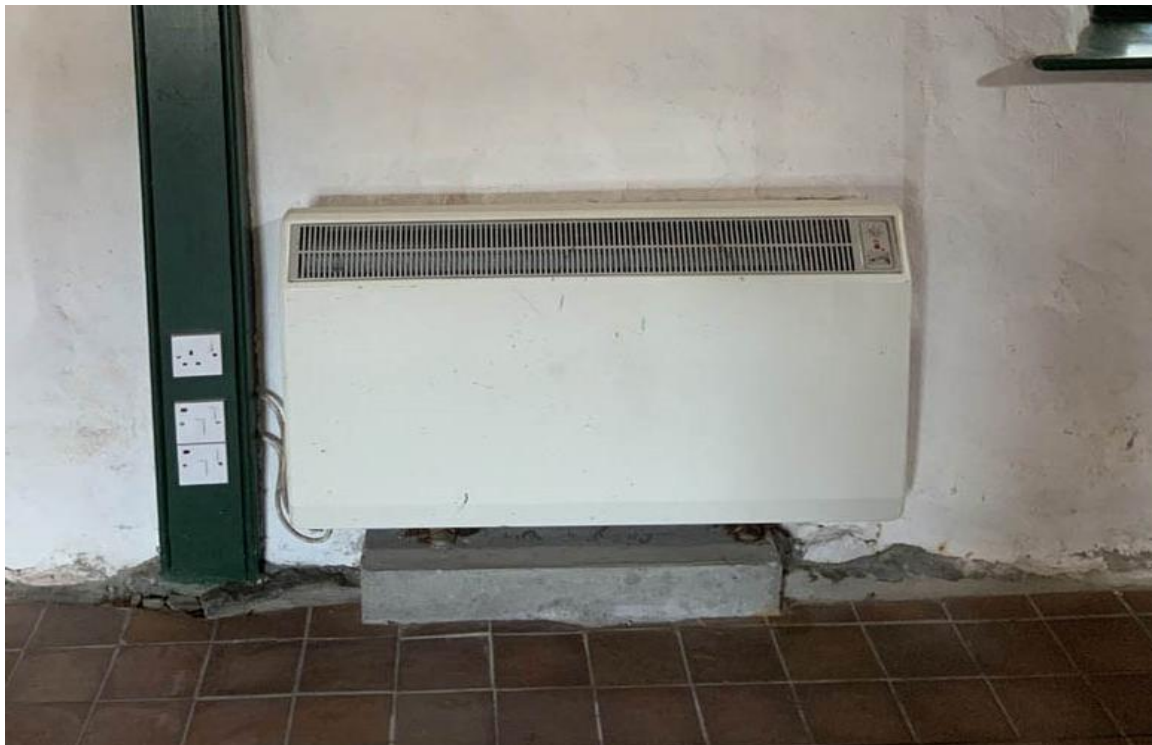
Image 20 – Example of current electric heater and surface mounted service run TO BE REMOVED
