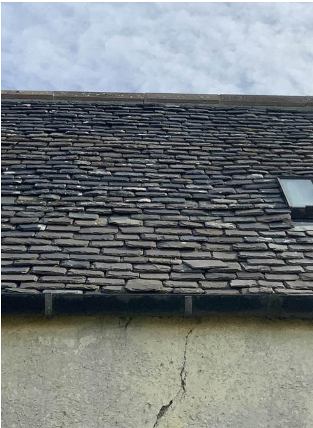
Image 8 – Existing Slate roof condition
