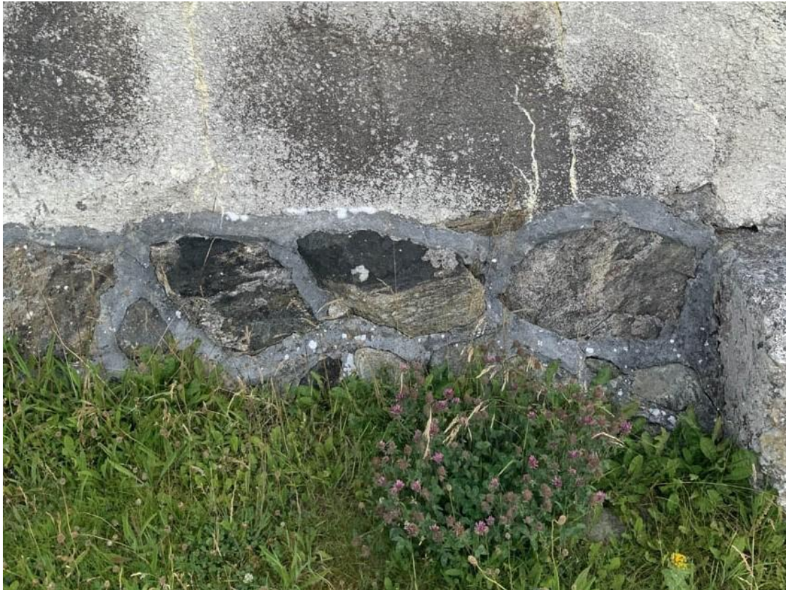
Image 19 – Example of Existing Cement Based pointing at ground level
