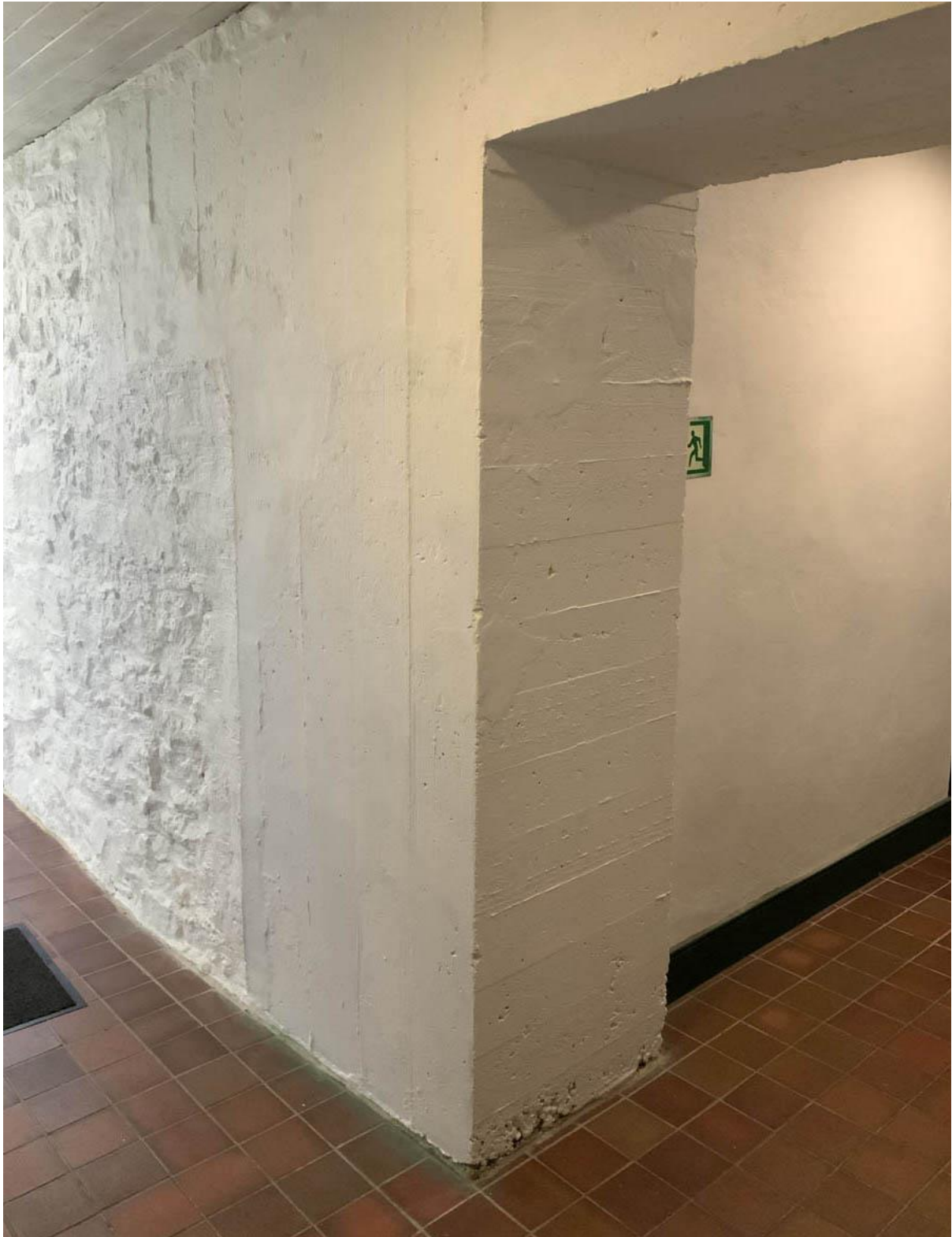
Image 14 – Existing painted internal opening formed in concrete (REF ID 13)
