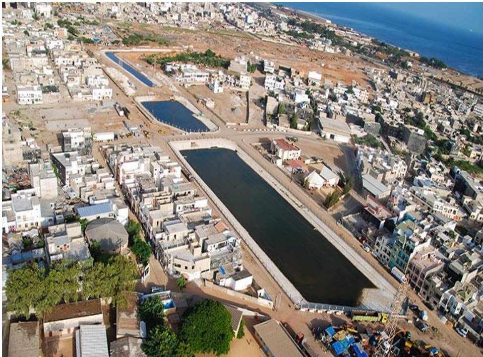
Reservoirs and drainage works built in Dakar to prevent flooding. © Agence de développement municipal (ADM)/PROGEP
