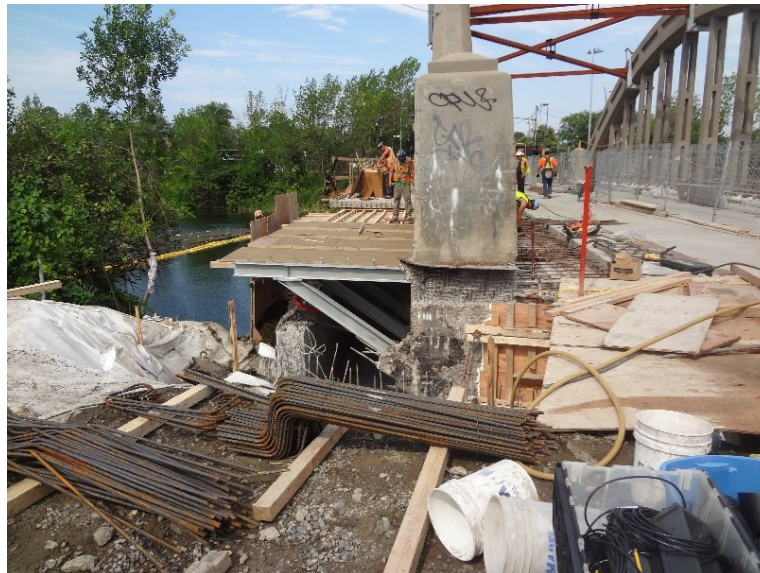
Figure 3.8 Project C; bridge side wall concrete casting project.
