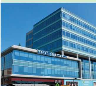
Rookwood Exchange Medical Office
