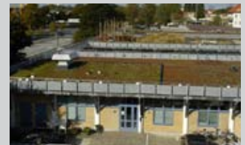
Green Roofs - Augustenborg Source: Jim Mueller, i-sustain.com
