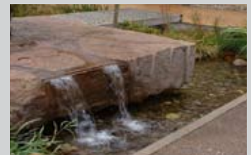
Stormwater management in Western Harbor creates a water feature in a central courtyard. Source: Dara O'Byrne
