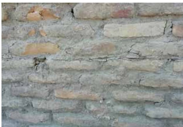
Water prevention layer between bricks.
