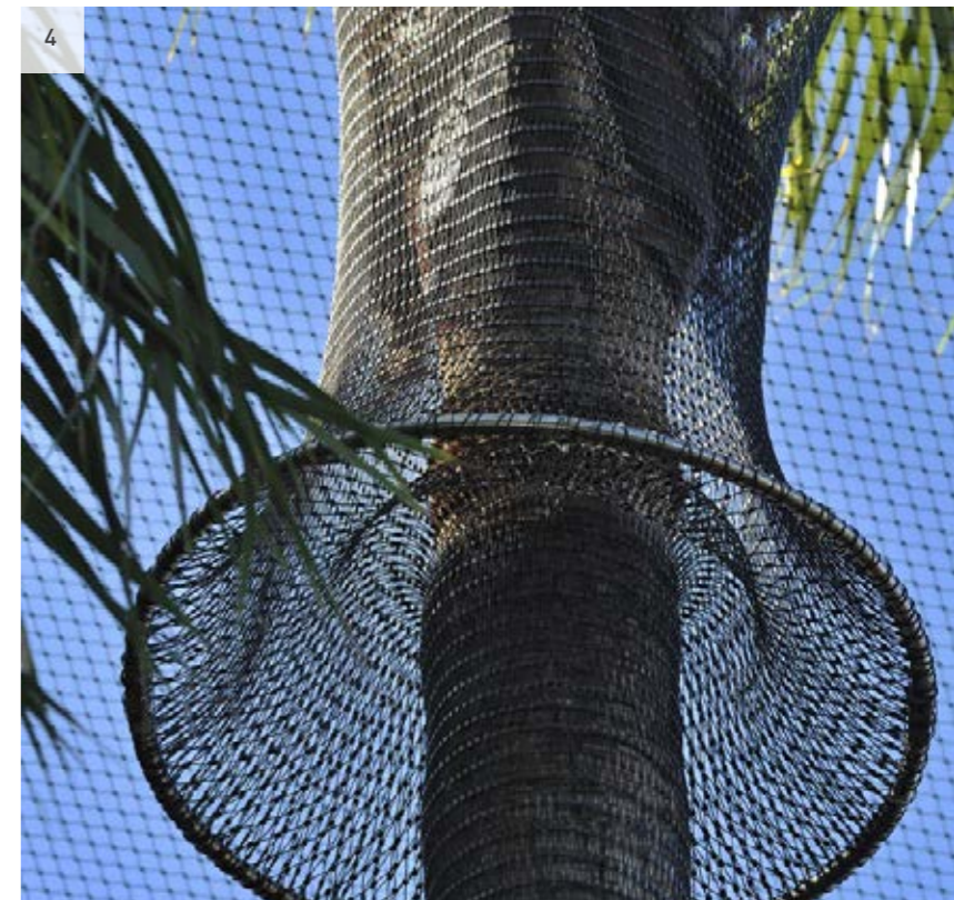
4 Mitwachsende Baumdurchdringung Size-adapting tree trunk penetration through the mesh
